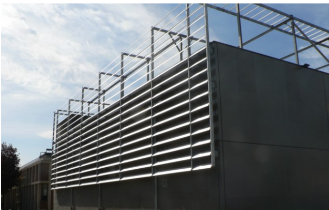
CC-IN2P3 new data center
